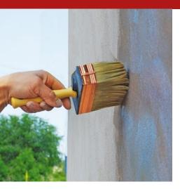
Reinforcing, fixative, transparent primer, based on stabilised potassium silicate for the preliminary treatment of the surfaces to be painted and/or plastered with silicate-based, lime putty, systems, for ecological building interventions, new buildings and for the restoration of vintage buildings and monuments.
