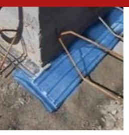
The SEALPVC SF 250 waterstop is a waterproof profile in PVC that is not hydro-expansive, having a thickness of 25 centimetres and high elasticity. It is used in static joints for horizontal casting (slabs), in concrete structures, resting on the substrate beneath the reinforcement.
