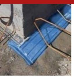
CUSTOMS CODE: 3925 9010 COMPONENTS: Single-component APPEARANCE: Extruded PVC AVAILABLE COLORS: Black / Light blu PACKAGING AND DIMENSIONS: Roll 20 m - Roll 25 m
