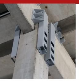
Two-component structural adhesive epoxy filler, with soft consistency, thixotropic, easy to spread (malleable paste), for the anchorage of steel connectors, the hermetic closure of through holes in concrete, bonding steel plates on concrete supports, as accessory product for laying road joints, for the reconstruction of wooden heads, crack repair, reconstruction of missing geometries, fixing injectors, reconstruction of joints in concrete floorings etc.
