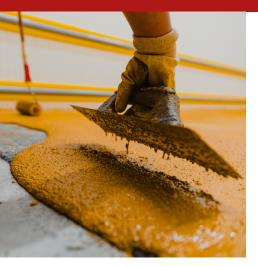
Two-component coloured, high solids, self-levelling and/or multi-layer epoxy coating on concrete surfaces and cementitious substrates.
