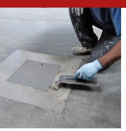
Syntech Grout EP is a solvent-free fluid epoxy mortar consisting of epoxy resins, special additives and selected aggregates of varying granulometry to restore structures in reinforced concrete, concrete paving, to create rigid joints, high-strength anchors and bar grouting. It is easily applied via simple pouring, to create layers of up to 5 mm in thickness.
