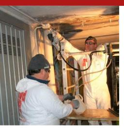
Mono-component semi-flexible, expanding (increases its initial volume of about 10 times) polyurethane resin, free from solvents, perfect for sealing small and large water leaks in the concrete or in solid masonry in general by injection. Perfect for filling and sealing small cavities, joints and discontinuities subject to movement.
