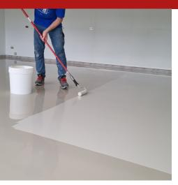
A 2-component coloured finish, with an epoxy resin base in aqueous dispersion. Ideal for the pigmented coating of industrial flooring and concrete products in general. Surfaces treated with Syntech Pavicrom are easy to clean and provide excellent resistance to mechanical wear, as well as having a high resistance to water, alkaline solutions, detergents and hydrocarbons (oils, diesel, petrol, etc.).
