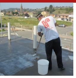
SYNTECH POLIUREA PRIMER - EPOXY is a two-component primer based on modified epoxy resins and special hardeners, solvent-free. Specially formulated to provide the right compromise between impregnation and wettability of the support to which, once applied, it forms a well-bonded layer.
