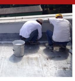
SYNTECH POLIUREA PRIMER-PUR is a single-component polyurethane primer with a base of low viscosity solvent, polyurethane resins and special isocyanates that, once applied, form an elastic film that adheres to the substrate. The processing times of this product range from 90 to 120 minutes, based on the percentage of ambient humidity.
