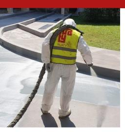
Syntech Poliurea Spray - FL is a pure polyurea designed for the specific application on driveways and parking lots in general. 100% solid does not contain VOC and can only be applied by spraying using suitable bimixer machines. It is characterized by a high degree of elongation. It is a coating elastomer obtained from the reaction of an aromatic type isocyanate with an amine.
