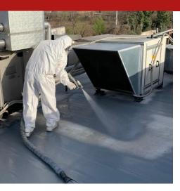
Syntech Poliurea Spray - N is a 100% pure polyurea of the aromatic type. It does not contain VOC and can only be applied by spraying using suitable bimixer machines which vaporise the material when hot. It is characterized by a high degree of elongation. Syntech Poliurea Spray -N is a coating elastomer obtained from the reaction of an aromatic type isocyanate with an amine. Both materials are extremely fluid and with low viscosity and have the property of reacting very quickly.
