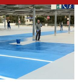
A protective, pigmented, two-component formulation based on aliphatic polyurethane resins, ideal as a protective and aesthetic coating on waterproofing with SYNTECH POLIUREA SPRAY. Characterised by high levels of elasticity and elevated protection, even in aggressive atmospheres. Available on request in shades from the RAL colour range.
