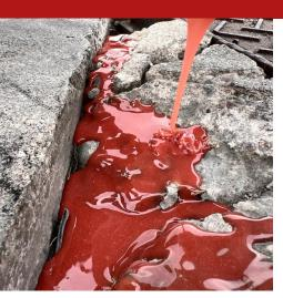
A fluid, medium-viscous epoxy adhesive for the structural casting of joints (new conglomerates on existing structures). After careful mixing, the two-component compound must be applied on the existing concrete by brush or roller, a few minutes before applying the new conglomerate ("wet-on-wet").
