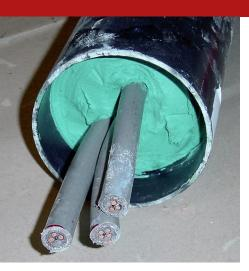
Mono-component Sealant compound, permanently plastic, slightly warm (+10% in volume in contact with water), for waterproofing underground holes, through which one or many wires and/or technical pipes pass, in masonry structures. It is extruded around the cables passing using specific dosing gun for 600 ml bags, and then covered with thixotropic mortar Repar Tix G2.
