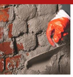
With the addition of mixing water only, this single-component premix creates a breathable, dehumidifying rough coating, preparatory to the application of restorative, dehumidifying, thermal-insulating and anti-condensation plasters, specifically Intosana, Sanatigh, Sanawarme and Caleosana, being plasters designed specifically for the healthiness of new buildings, existing buildings, works on green buildings and in the restoration of historic and monumental buildings.
